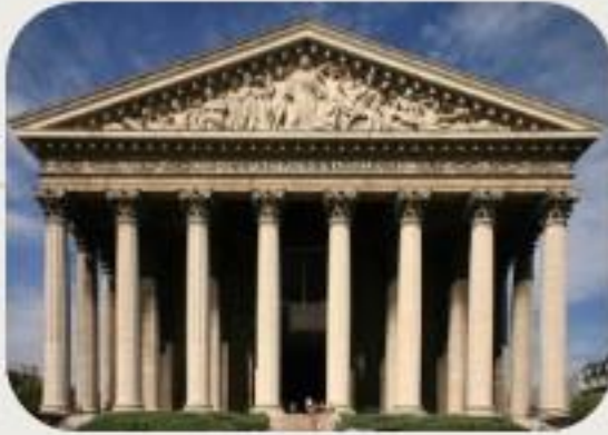
Tall columns that rise the full height of the building
